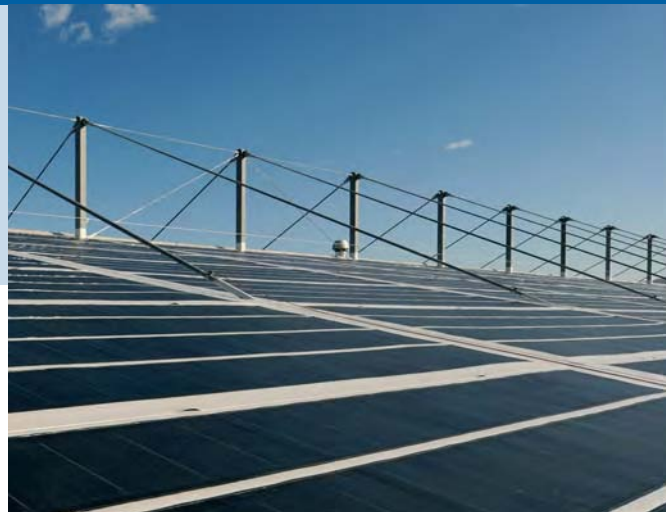
Fig. 2 - Grödenmoos Stadium. Switzerland's largest solar power plant with an installed capacity of 56 kWp made of roofing membrane with integrated thin-film photovoltaic cells. The Grödenmoos Stadium in St.Gallen is the venue of the international CSIO horse riding competition in Switzerland. Surface: 1 200 m². Owner: Sankt Galler Stadtwerke (photo energiebüro, Switzerland).
