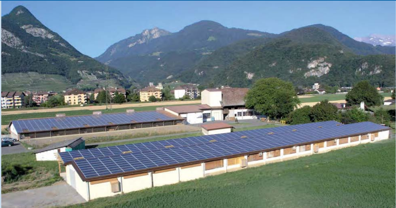
Fig. 1 – La Ferme des Trois Epis, Aigle (VD). This chicken farm has an integrated system with 160 kWp solar tiles "oryon" (Solar Fabrik cells) and Swiss inverter SolarMax 80C (2 units); by Solstis, Switzerland (photo Solstis, Switzerland).
